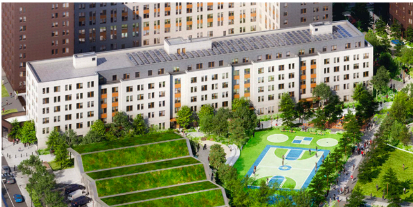
Alafia Building C3 Completion by December 2024 Brooklyn (East New York), NY
