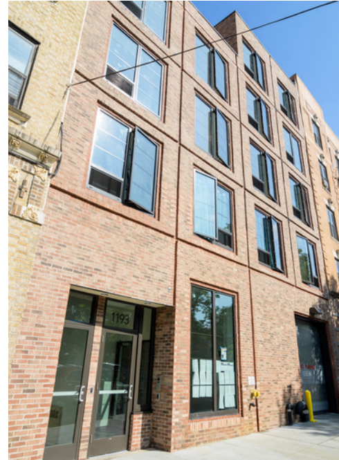
1193 Fulton Ave, Bronx. Completed in May 2022.
